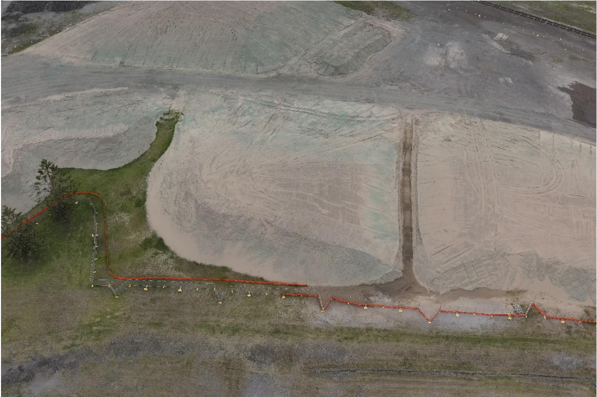
Photograph 1: View of Outer Harbour stockpiles following polymer application and sediment controls.
