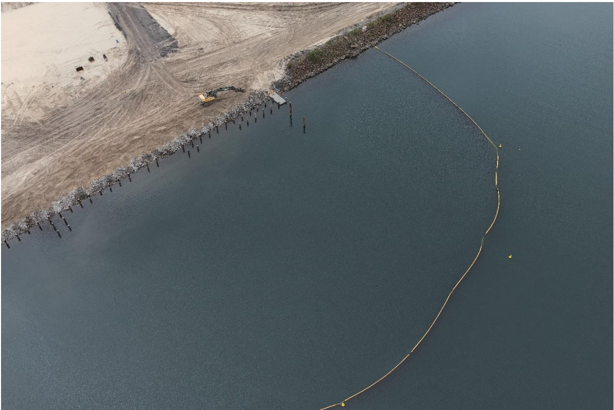
Photograph 2: View of removed wharf apron and remaining wharf piles at Berth 101.
